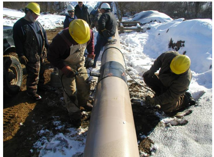
Application of Dirax Sleeve
