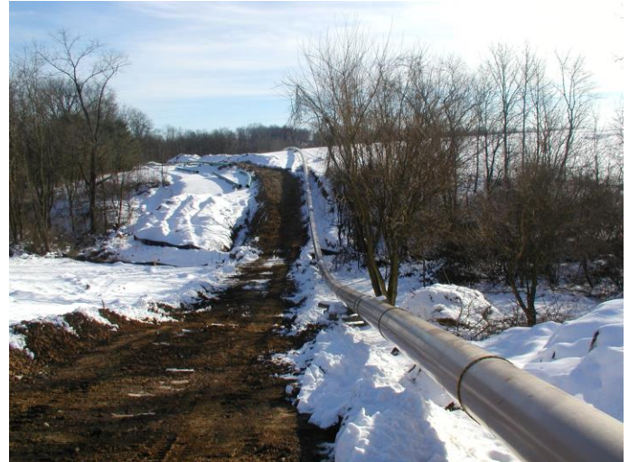
Job Site Overview
