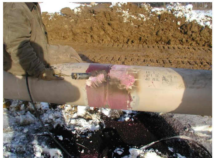
Removal of Liquid Epoxy System
