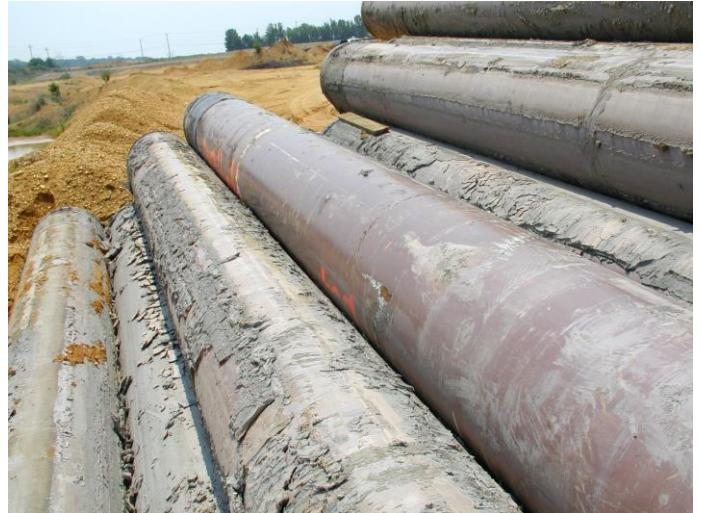
Recovered Directional Drill Pipe
